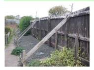
Station Cottages - - Work has been completed to stabilise the highway and to build a retaining wall along the front of Station Cottages to stop future problems of landslip into their gardens and subsidence of the road. As can be seen in the "before" and "after" photos the result is dramatic.
